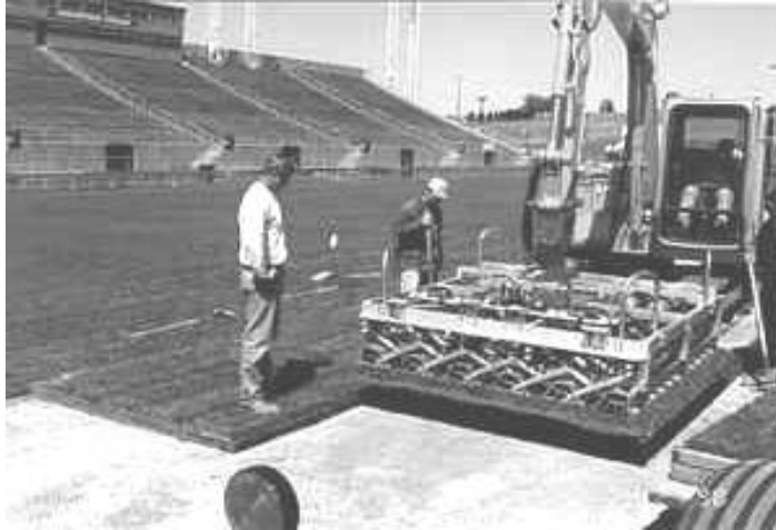
Fig. 3. Tile being installed over sand base.
