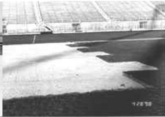
Fig. 2. Area prepared for tile installation.
