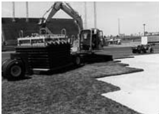
Fig. 1. Removing tile from container.
