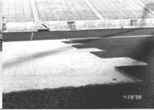
Fig. 2. Area prepared for tile installation.
