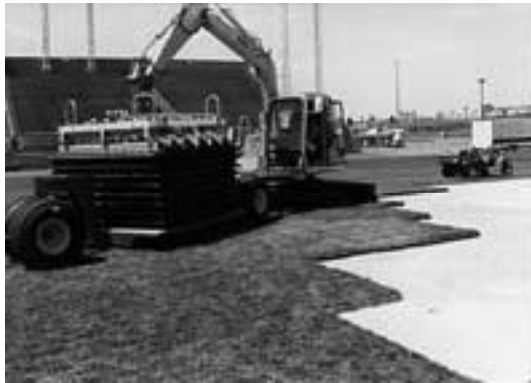
Fig. 1. Removing tile from container.
