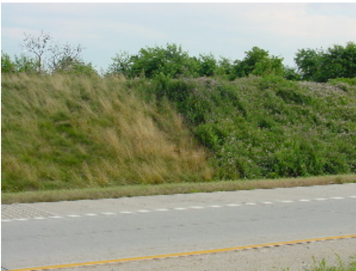
Figure 2. The grass-based Formula L (l) and crownvetch (r) are shown growing side-by-side on a soil berm. Crownvetch will grow on harsher sites than Formula L, but on sites such as this the grass-based formula provides a low-growing, densely rooted cover that is easier to keep free of broadleaf weeds by using selective herbicides.
