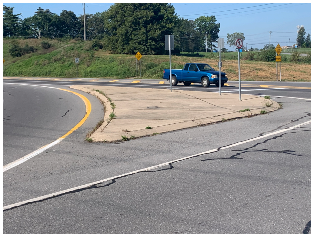
Figure 2. A traffic island that will be spot sprayed with a handgun application to provide total vegetation control. Herbicides used for these applications shall provide label directions allowing for spot treatment, crack and crevice, or "hardscape" applications.
