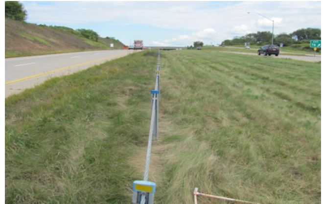
Figure 6. Cable guiderail with low growing fine fescue groundcover maintained with regular mowing up to cable guiderail plus broadleaf weed control applications.
