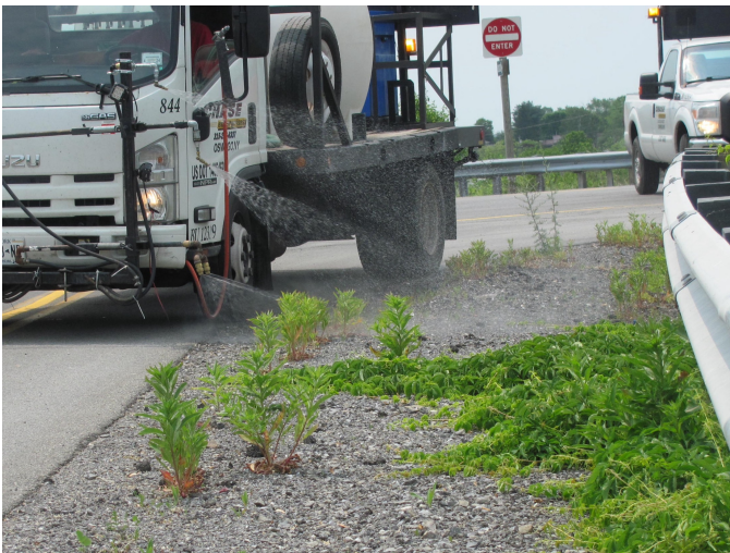
Figure 1. Most total vegetation control applications to roadsides are fixed-pattern, truck-based treatments to guiderails, concrete barriers, and shoulders. Signposts and traffic islands are treated with a handgun application.
