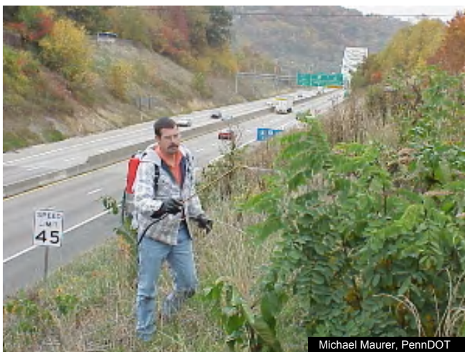
Figure 6: A selective application of an herbicide mix to roadside brush. The backpack sprayer with a nozzle that delivers a small volume of spray solution is well suited to selectively treating target weeds and leaving the desirable groundcover uninjured.
