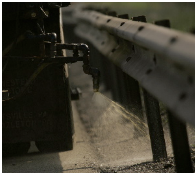
Figure 1. Most total vegetation control applications to roadsides are fixed-pattern, truck-based treatments to guiderails, concrete barriers, and shoulders. Signposts and traffic islands are treated with a handgun application.
