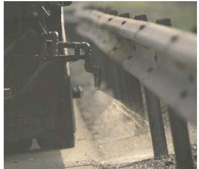
Figure 18. A non-selective herbicide mixture is applied to a highway guideway to prevent weed growth. Herbicides in the mixture eliminate existing growth and prevent establishment of new weeds from seed.
